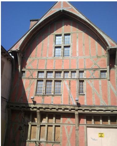
The advantage of this technique is to allow the rapid construction of buildings of several levels at a lower cost than stone buildings. The necessary materials were available locally: wood for the framing, mortar made of earth or an assembly of terracotta bricks for filling and stones for the basement.
